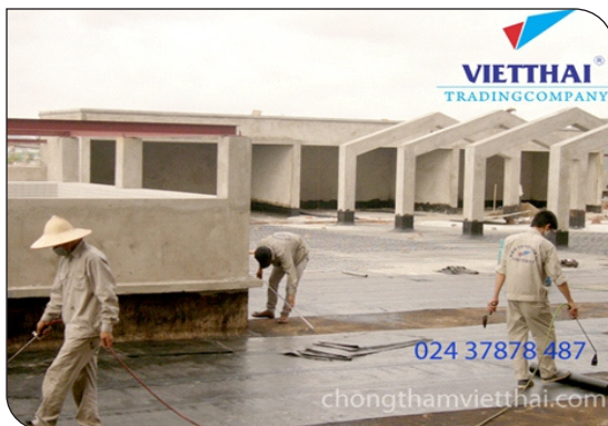
Construction of torched on membrane
